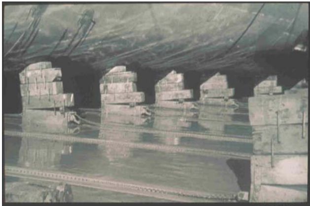
SLIDING RELEASING BILGE BLOCK
