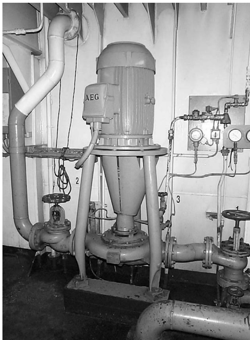
Figure 12 A vertical electric-driven centrifugal water pump
